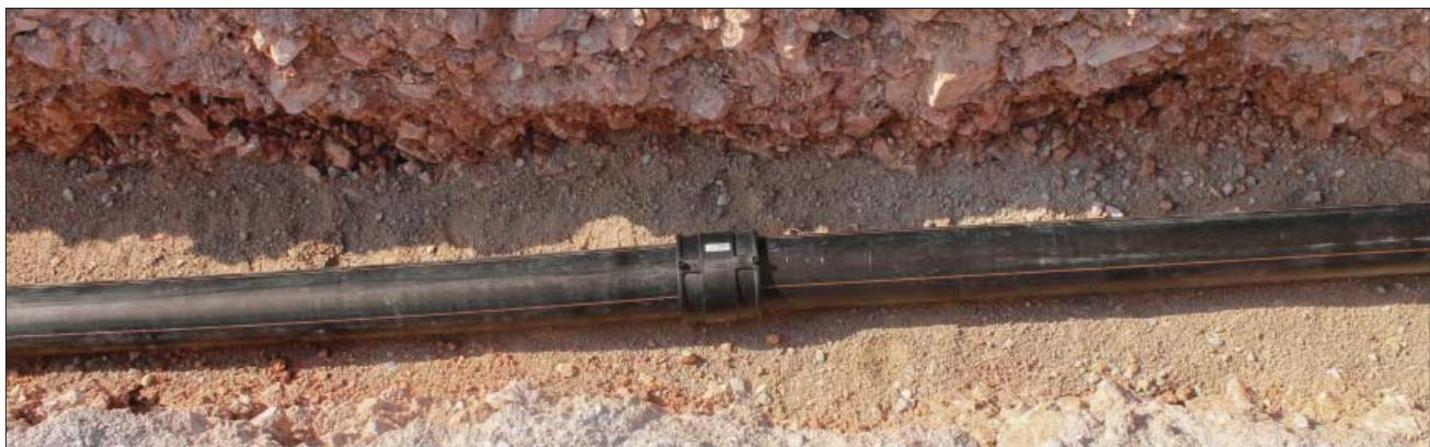
Mechanical fittings are limited to smaller pipe diameters, and are mainly used for water supply.
