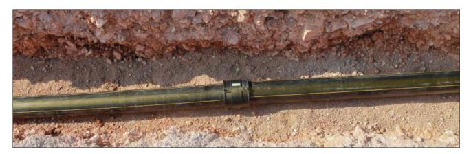
Mechanical fittings are limited to smaller pipe diameters, and are mainly used for water supply.
